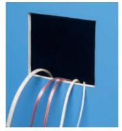
1 Determine box location. Cut hole. Pull wire and cable(s) through appropriate knockout (connector).
